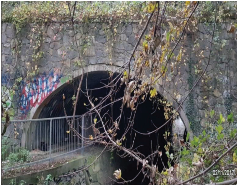
Figure 12: B31 Blanchardstown Bypass Bridge 1
